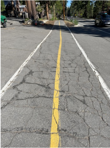
Alligator cracking
