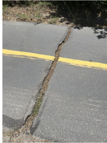
Transverse cracking
