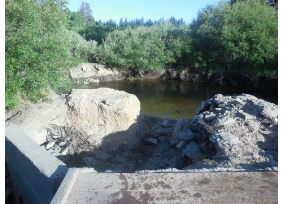
Summer 2017, bridge not connected to West side
