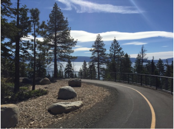
Meeks Bay Trail Completed
