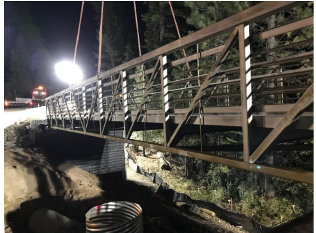
Meeks Bay Trail bridge construction
