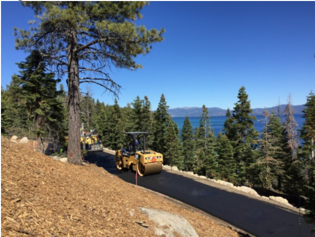
Meeks Bay Trail Construction Paving
