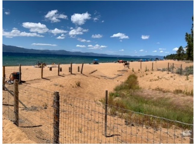
Nevada Beach enclosure before maintenance.
