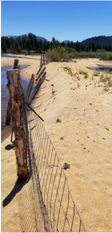
TYC fencing in need of repair at Baldwin beach 2021
