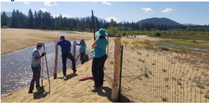
Volunteers rebuilding fencing at Baldwin Beach, 2021
