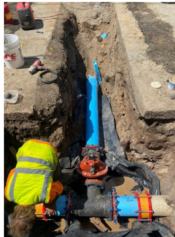
East project watermain tie-in location @ Martis Peak intersection w/Crystal Peak
