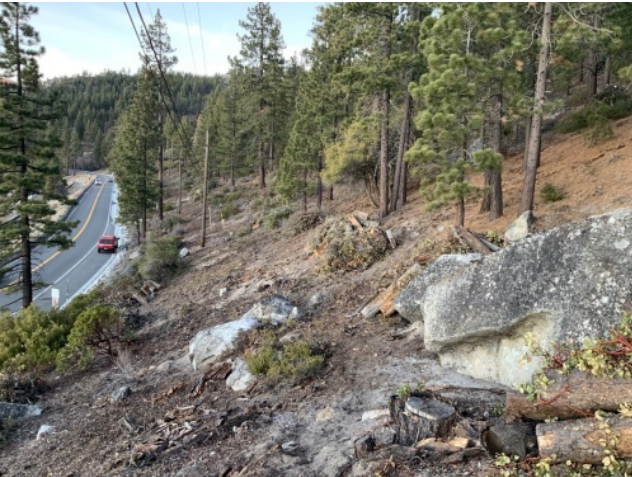
Finished fuels treatments along Incline 4100, near Sand Harbor
