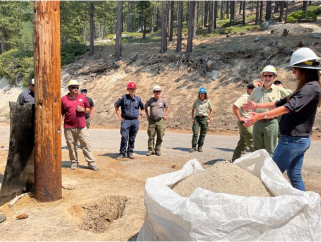
NV Energy host site visit at an active pole replacement site at Ponderosa Ranch. Picture shows the existing pole and replacement hole and excavation materials bagged for replacement.
