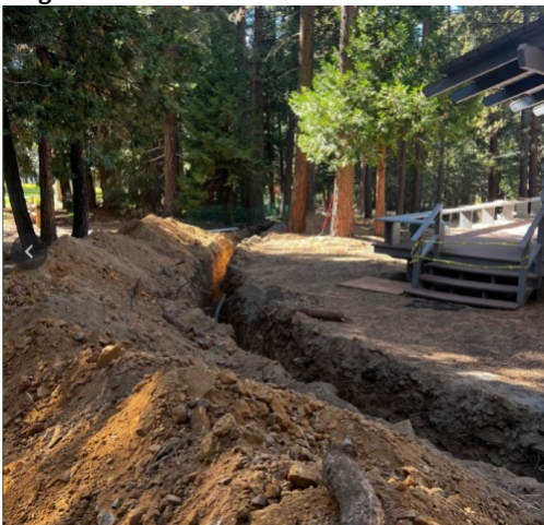
Undergrounding of utility lines
