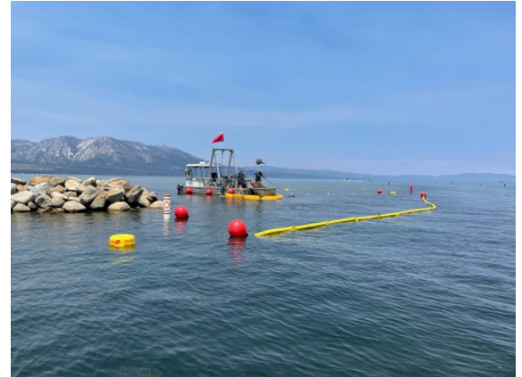
Dive team offshore of the West Channel of the Tahoe Keys implementing diver-assisted suction removal.
