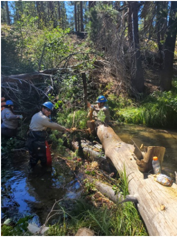
CCCs building a LWD structure in Trout Creek
