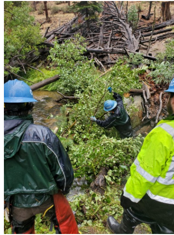
CCCs building a post assisted log structure in Trout Creek
