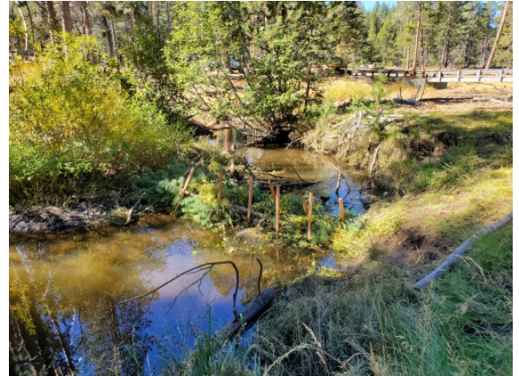
Completed Post-Assisted Log Structure
