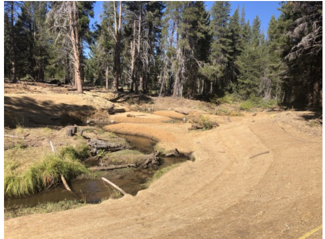
October 2022_Completed project looking downstream
