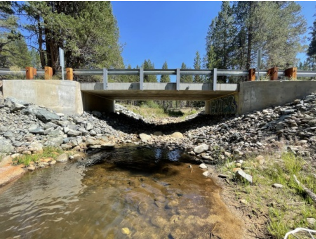
Completed bridge replacement_2018
