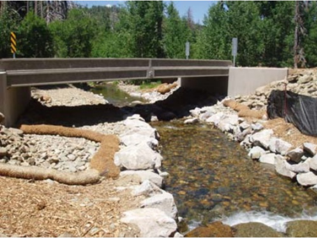
a new bridge replaced an undersized, failing culvert at Spring Creek Road
