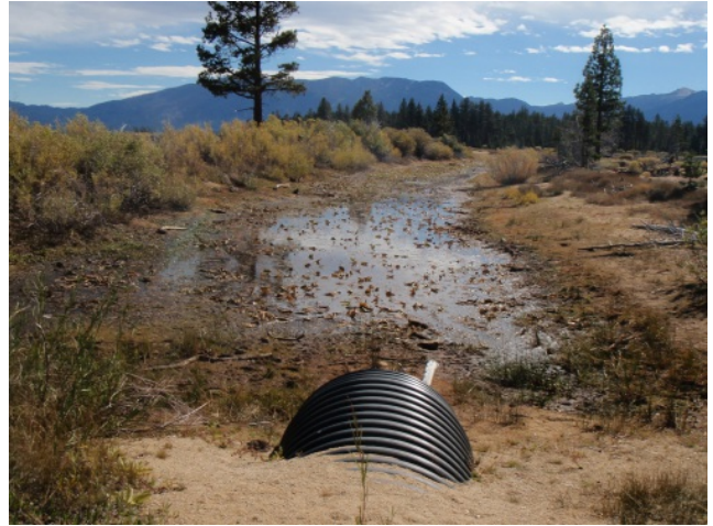
Existing Beach Access/Culvert Dissecting Swale 1
