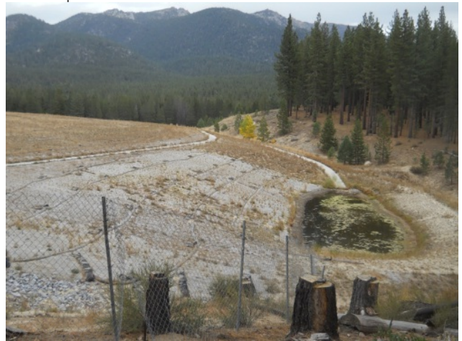
2- Southern End of Landfill with Drainage Features
