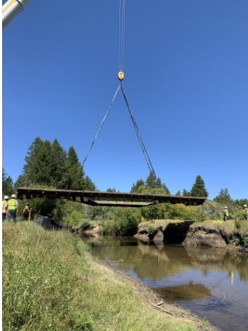
Temporary bridge crossing Upper Truckee River
