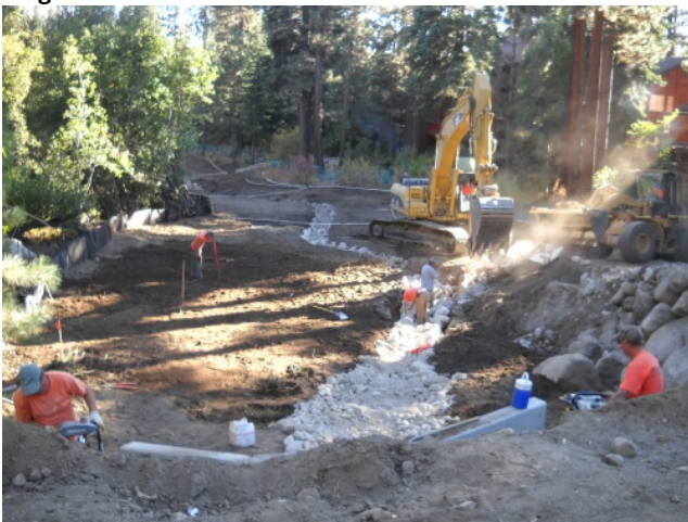
Construction of channel and floodplain Sept 2012
