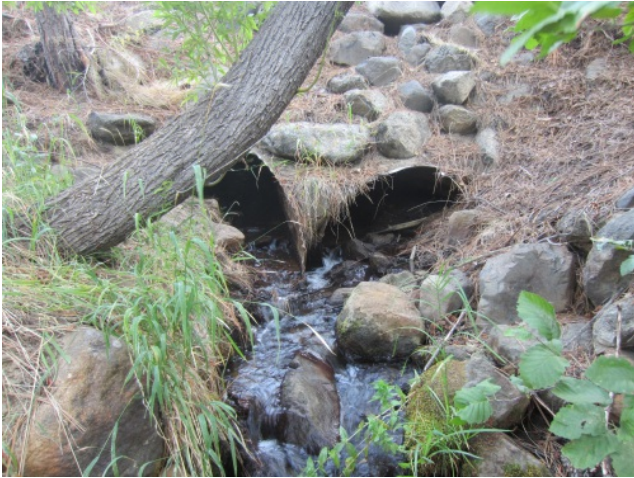
Culverts below Northwood before construction
