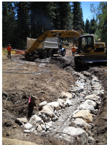
Building channel and floodplain Sept 2012
