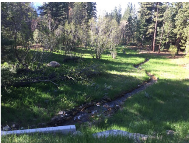
Post construction May 2016
