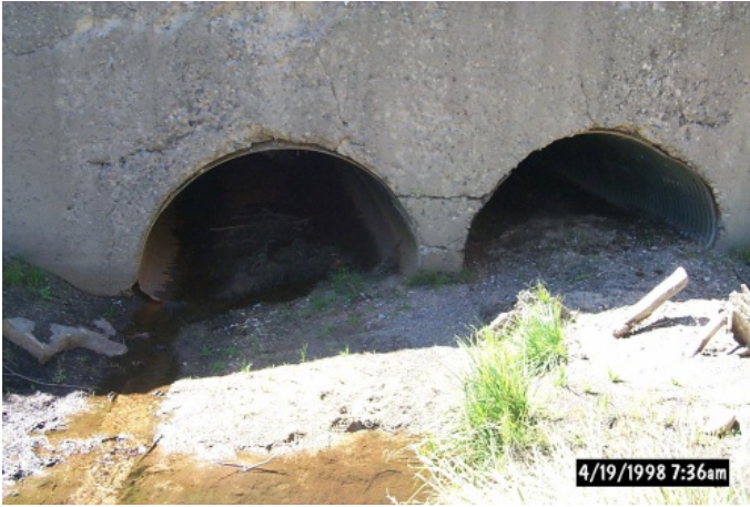
old, impassable culvert on Angora Creek at Lake Tahoe Blvd
