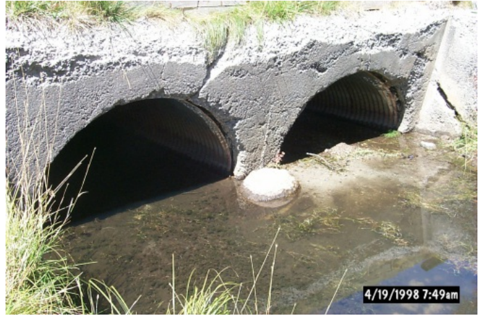
old, impassable culvert on Angora Creek at View Circle
