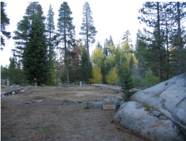
Site of demolished caretakers house
