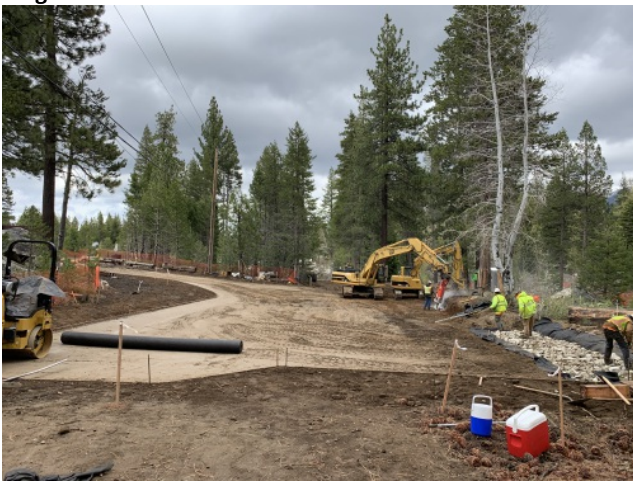
Parking lot construction
