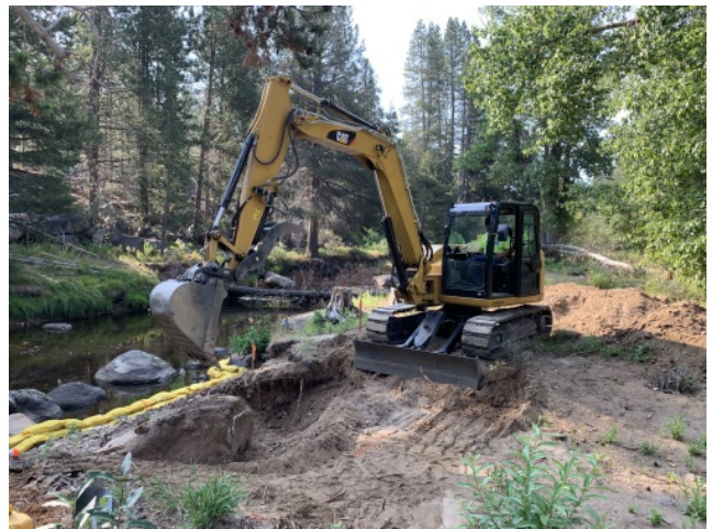
Swale inlet construction
