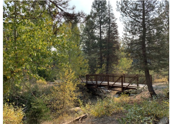
New bridge on path to Upper Truckee River
