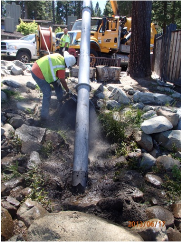
Telecoping boom extended and rodder hose during operations
