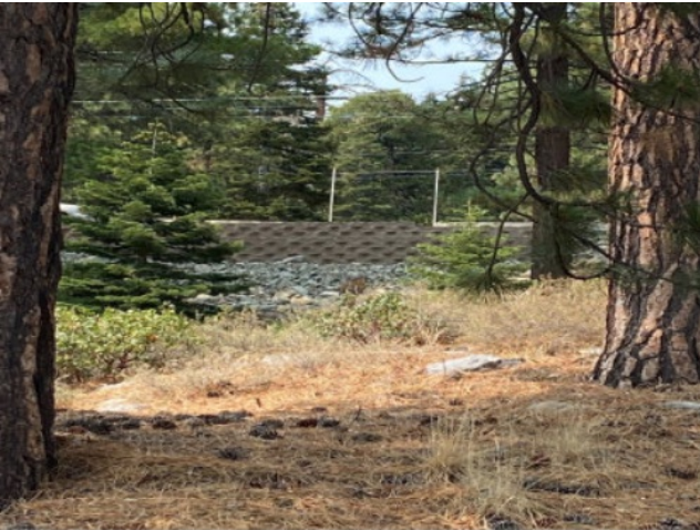
New Beowawie retaining view - view from below
