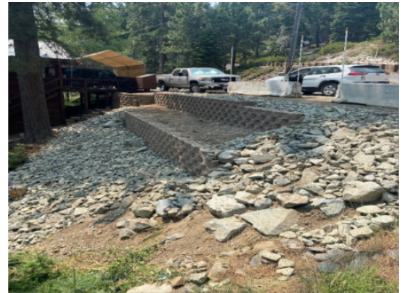
Completed Beowawie retaining wall from street view
