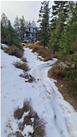
runoff creating erosion on USFS parcel onto NDSL parcel
