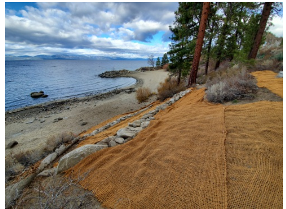
Cave Rock hillside erosion control measures
