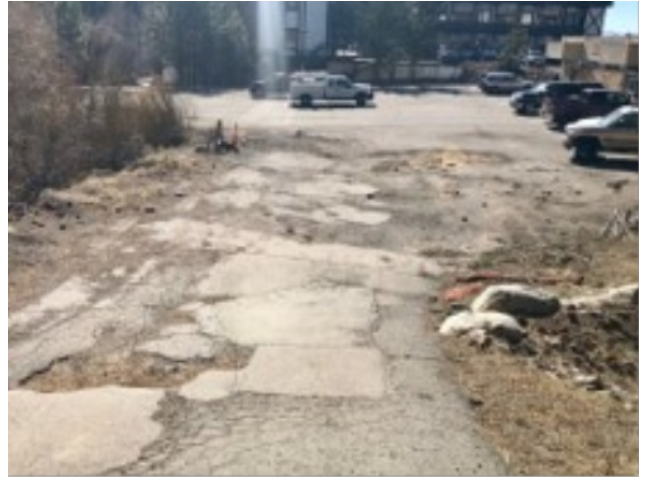
Degraded asphalt and lack of parcel BMPs adjacent to the Edgewood Creek Tributary
