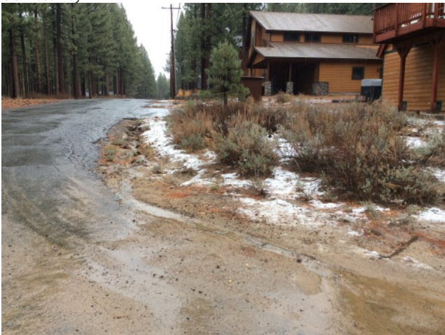
Road shoulder erosion (Red Lake Road/Walkup Road)
