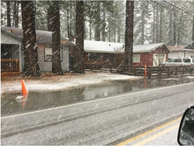
Inadequate road drainage impacts ability to use achieve TMDL Road RAM scores - Glenwood Way
