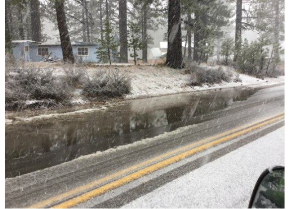
Road condition impacts from inadequate drainage and need for source control - Glenwood Way
