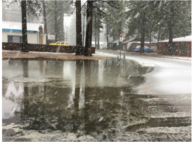
Inadequate road drainage and road shoulder stabilization - roadway flooding impacts ability to achieve TMDL Road RAM scores
