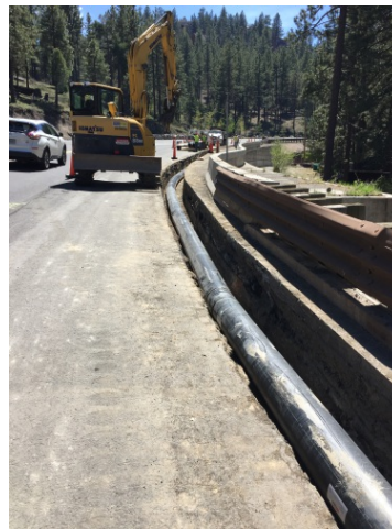
Installation of 950 feet of stormdrain pipe
