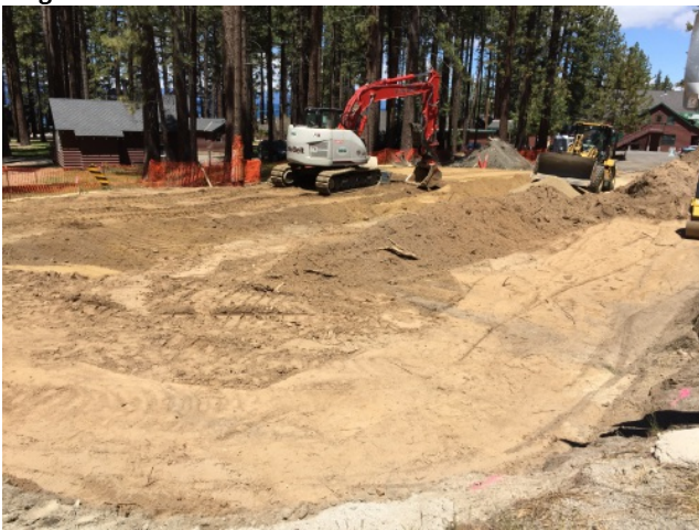
Construction of a 8500 cf infiltration basin
