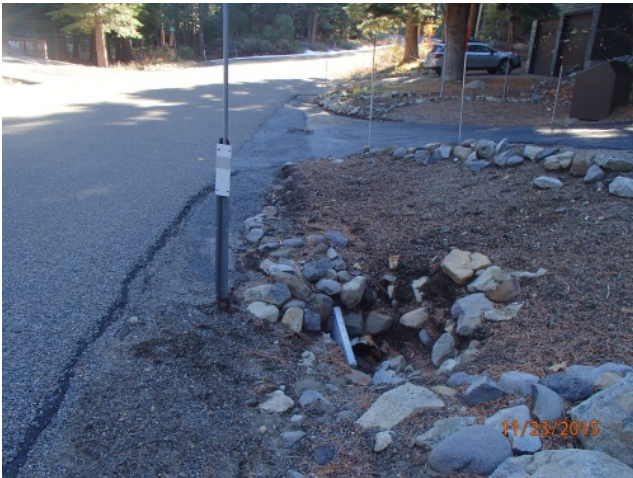
Partially buried pipe inlet(s) on Antelope. Opportunity for Sediment Trap to increase inlet and trapping capacity.
