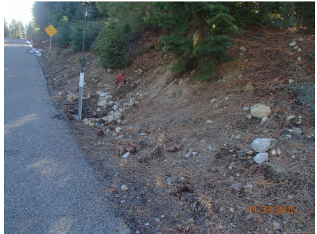
Eroding slope near pipe inlet
