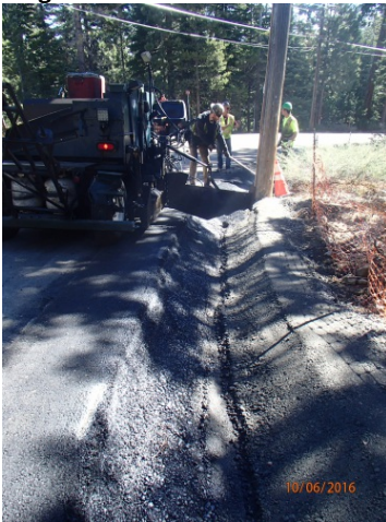
Construction of AC swale on Antelope Way
