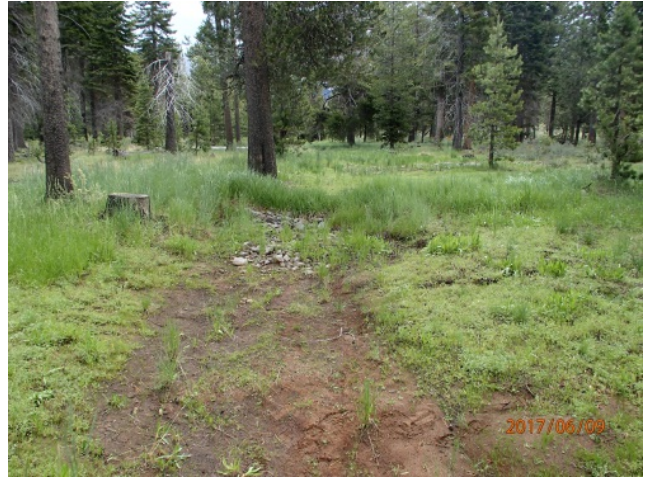
Previously constructed water quality improvement project near Pioneer Tr & US Hwy 50.
