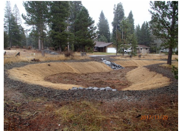
Completed infiltrating sediment basin.
