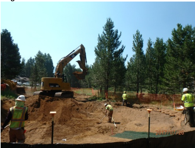
Construction of infiltrating sediment basin.
