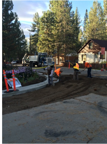
Curb & Gutter and Drainage Inlet Construction
