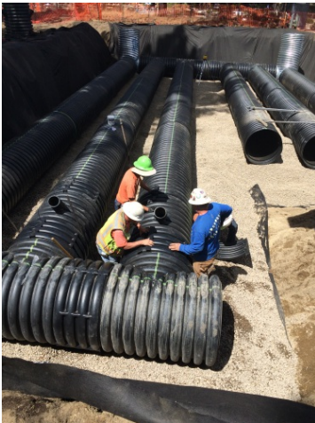
River Street Infiltration Gallery - under construction
