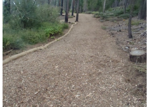
Decompacted & Recontoured NFS Rd North of Boulder Mt. Road
