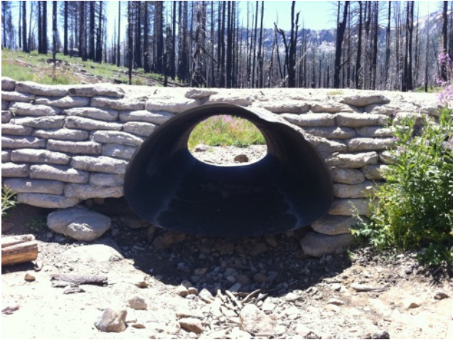
Squash Culvert Before Removal / Restoration
