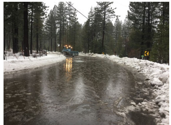
2016- Inadequate drainage creates flooding on South Avenue (major access road to Barton Hospital)
