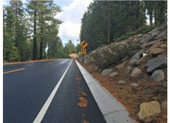
Rock slope stabilization and gutter pans added to sections of Highway 89 between Meeks Bay and Emerald Bay
